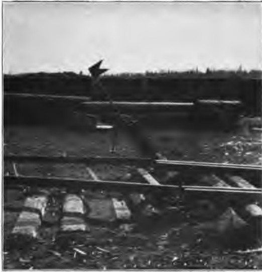
ATLANTIC MINE. No. 3.—Switch Stand Shown on Right Edge of Plate 2. Shows Turning of Ties Caused by Movement of Rails.
